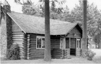
Adair House in Anderson Park
